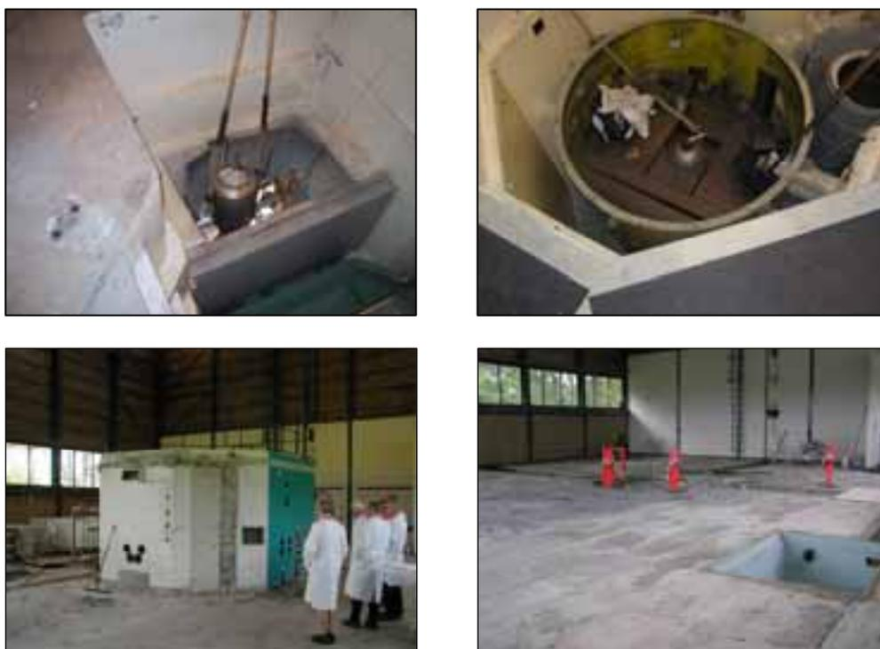
Figure 2. (Upper left) removal of the recombining, (upper right) removal of graphite and the reactor core, (lower left) biological shield after removal of control rod housing, (lower right) biological shield removed.
