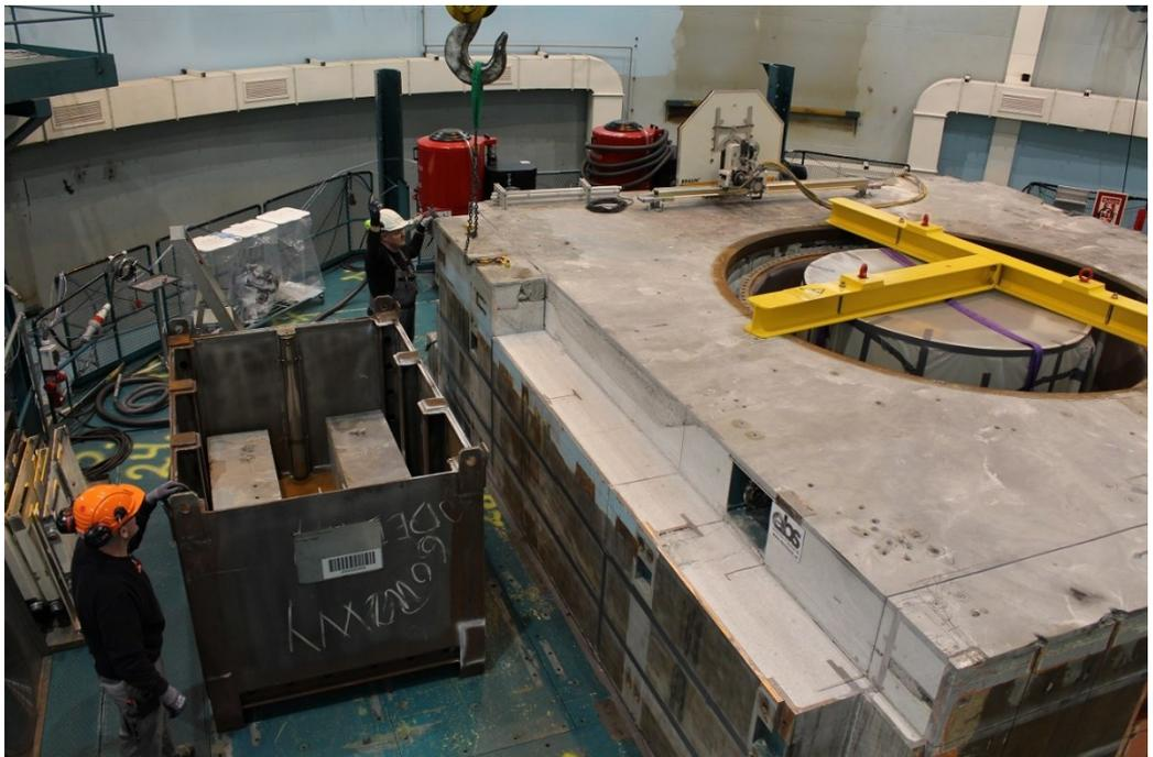
Figure 5: Lifting of one of the cut blocks to a DD type 2 steel container
