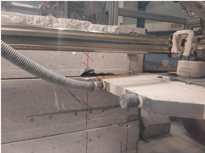
Figure 8: Challenges with the circular saw cutting in a mix of concrete and steel
