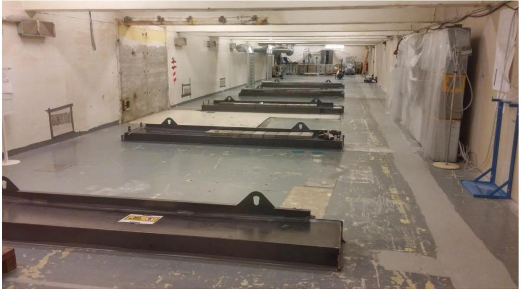
Figure 12: Dummy shutter housings with dummy shutters on the top surface of the row of hot cells, before modification.
