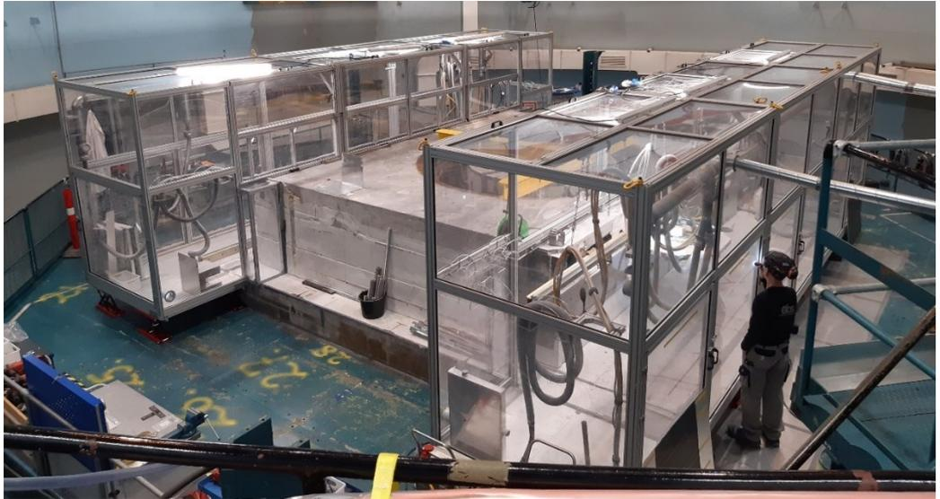
Figure 4: Dust containments mounted on facade 1 and 3. Ventilation ducts for the dust containments are connected to the vacuum extractors at the ground level.
