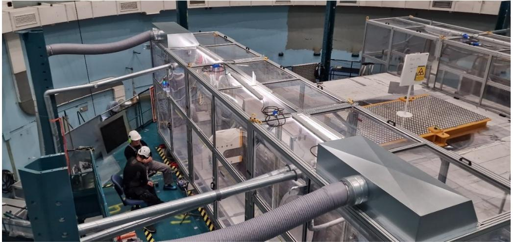
Figure 7: The new recirculation of the ventilated air in the dust compartments.
