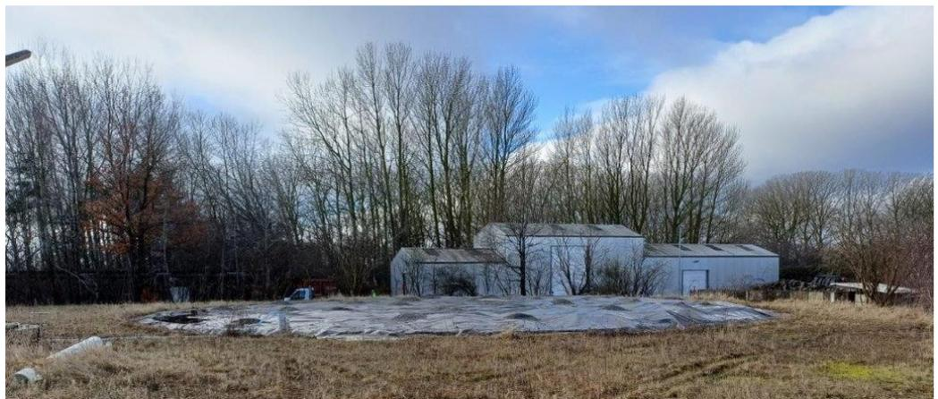
Figure 31: One of the basins with cover with heavy-duty tarpaulin material
