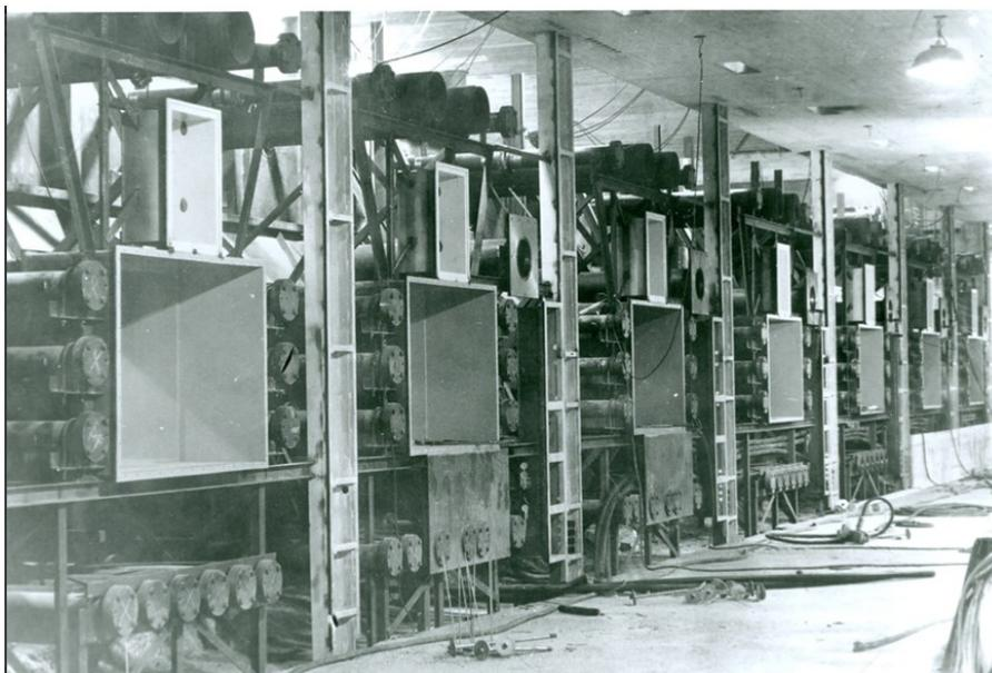
Figure 11: Picture from the construction of the Hot Cell Facility in the 1960's showing some of the now embedded cables and tubes.
