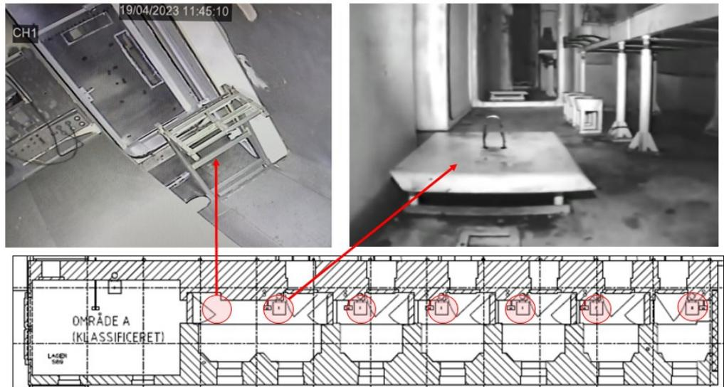
Figure 21: Steel rack and ventilation filter covers in the hot cells
